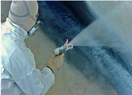
Paint protector of electromagnetic radiation. It is applied to protection against electromagnetic radiation (Germany)
